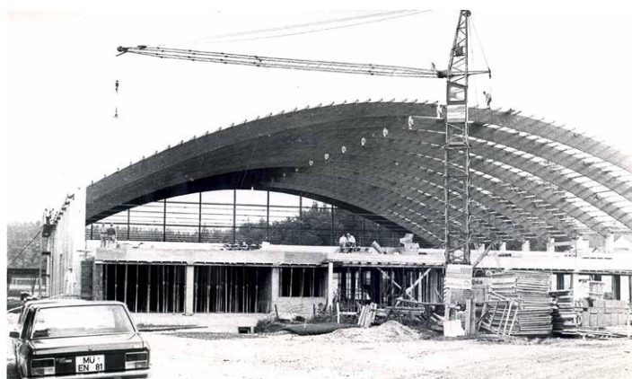
Eissporthalle in Bau, Sommer 1975.
